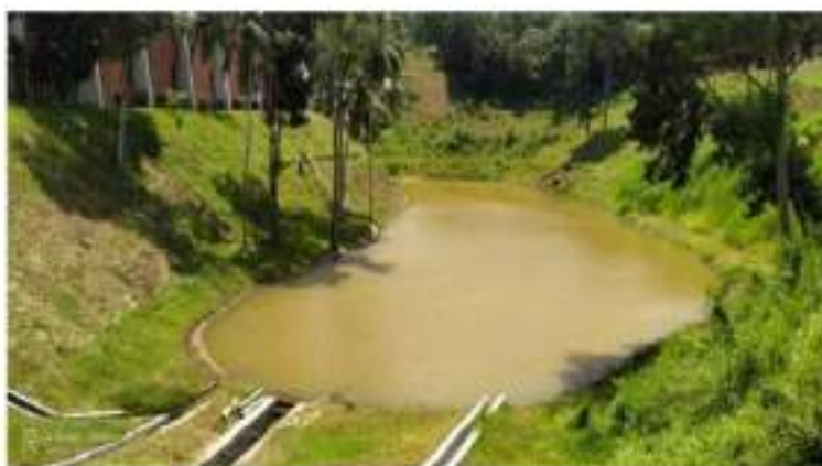
Rain Water Harvesting
